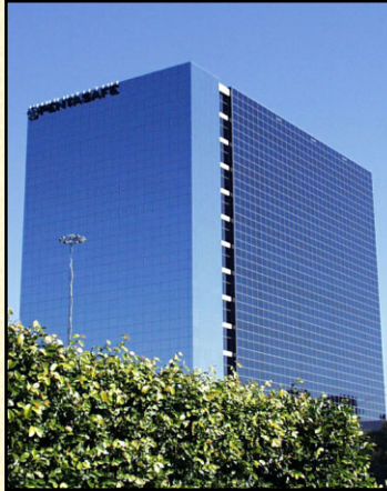
PENTASAFE, INC. PARK TOWERS OFFICE COMPLEX HOUSTON, TEXAS
